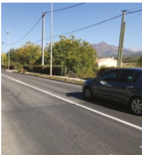
Development of Digne-les-Bains feeder road
