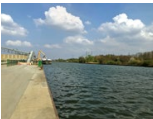
Maintenance dredging on Rhone-Rhine canal
