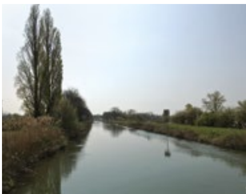
Maintenance dredging on Rhone-Rhine canal
