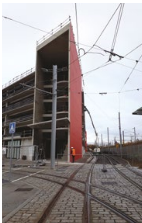
Euro3Lys project in Saint-Louis
