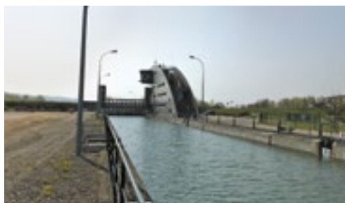
Maintenance dredging on Rhone-Rhine canal
