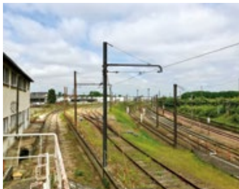
Orléans - Châteauneuf-sur-Loire railway line
