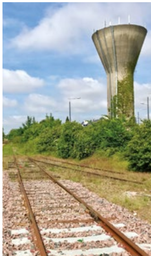
Orléans - Châteauneuf-sur-Loire railway line
