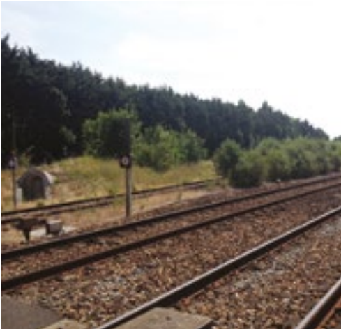
Electrification of Amiens - Abbeville - Rang-du-Fliers rail link
