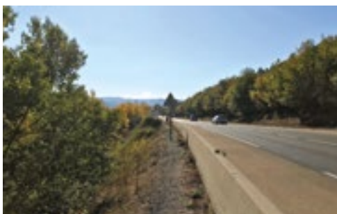
Development of Digne-les-Bains feeder road
