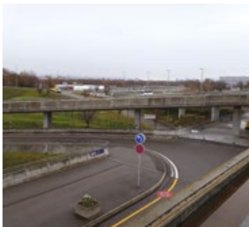
Euro3Lys project in Saint-Louis
