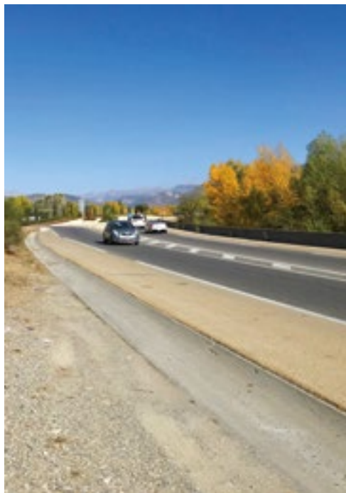
Development of Digne-les-Bains feeder road
