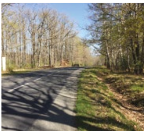
Sansac-de-Marmiesse (national road RN 122) by-pass
