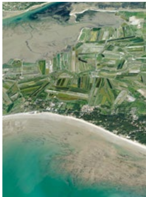
La Couarde-sur-Mer dyke reinforcement project
