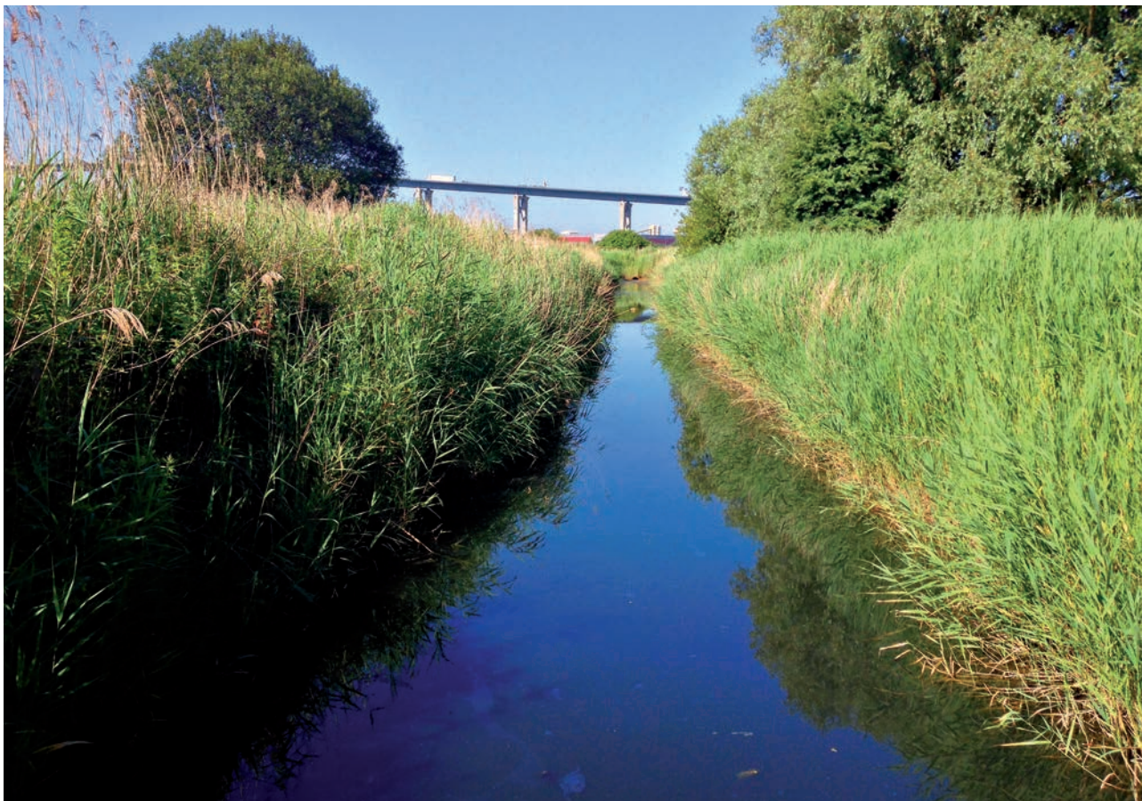
# MAJOR SOUTH-WESTERN RAIL PROJECT (GPSO): NEW BORDEAUX LINES
