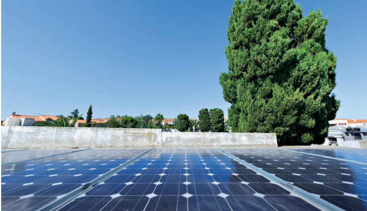
# ENERGY-COMPENSATED INSTALLATION TO LIGHT THE ST JULIEN CHAPEL IN VILLENEUVE-DE-LA-RAHO
