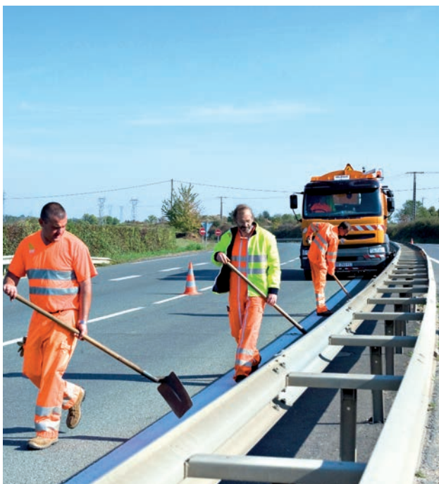
# DIR WORKERS ON THE RN 174 NORTH OF POITIERS
