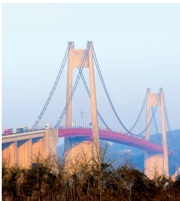
# VIEW OF THE TANCARVILLE SUSPENSION BRIDGE CROSSING THE SEINE BETWEEN TANCARVILLE AND MARAIS-VERNIER
