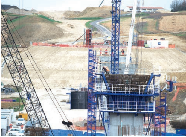
# SUD-EUROPE-ATLANTIQUE HIGH-SPEED LINE: INSTALLING THE FIRST VOUSOIRS IN THE BOËME VIADUCT
