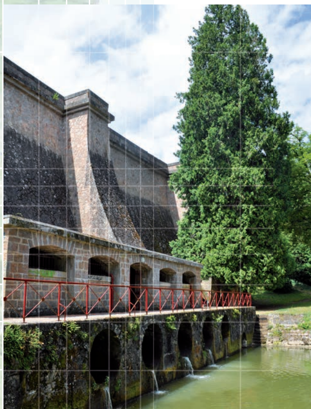
# RENOVATION OF THE PONT-ET-MASSÈNE DAM
